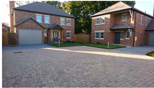
Figure 1: Example of Permeable Driveways
